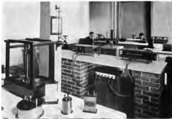
A Working Corner in the Standard House
